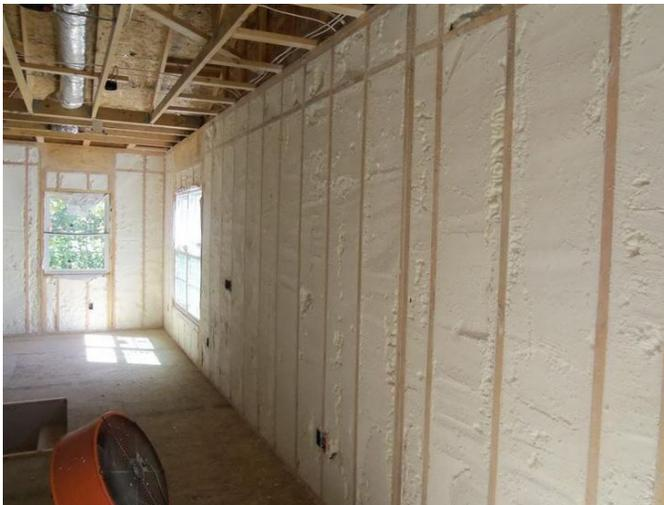
**Closed Cell 2 lb. Foam** –Excellent Insulating Properties. Closed cell 2 lb. foam is sprayed onto walls as a liquid before expanding into a hard foam. Closed cell foam is completely air tight, moisture proof, guaranteed for the life of the home owner and actually adds strength to the building it is installed in.
